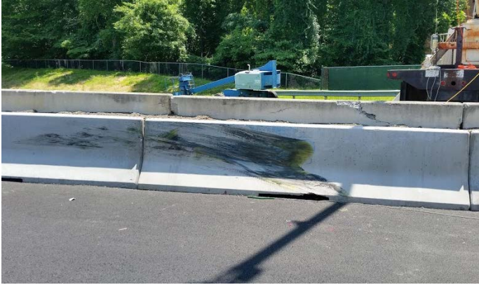
The jersey barrier after impact. Photo credit: FHWA
