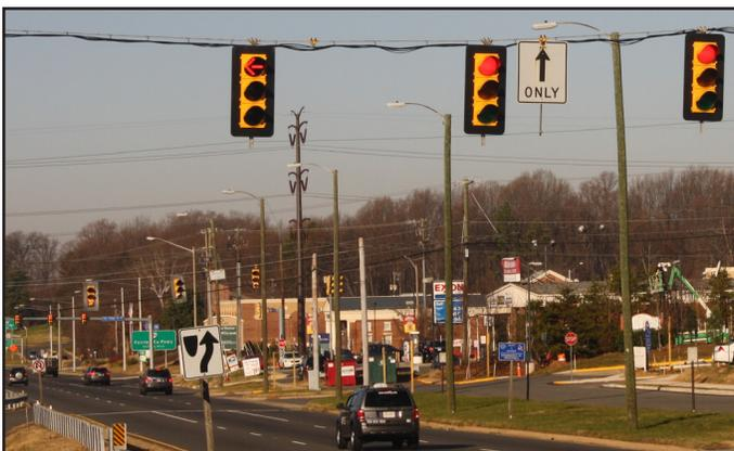
Exhibit 12: Example of closely spaced signals. (Source: VHB)
