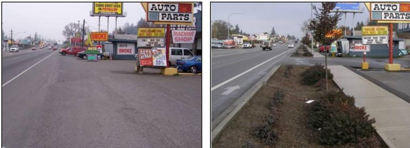
Exhibit 1: Washington State Department of Transportation (WSDOT) conducted an analysis of the crashes in the corridor before and after the measures were in place. The results of the analysis showed that implementing access management practices significantly reduced accident severity and societal costs. (Source: WSDOT)
